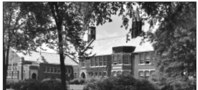
View of Howard School, which is featured in "Lost Wilmette," the current exhibit in the lower-level gallery of the Wilmette Historical Museum at 609 Ridge Road.
