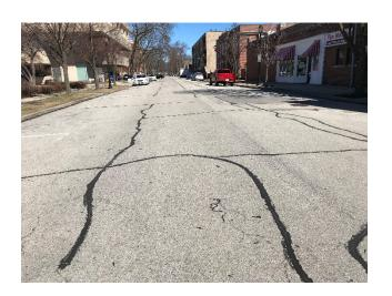
Crack sealing is the second stage of the pavement maintenance program. The purpose of this project is to seal cracks that have developed or expanded on surface of asphalt-paved streets. The goal of this product is to prevent moisture from reaching the base and increasing the rate of pavement degradation.
