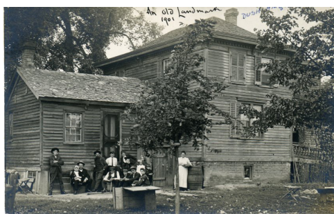
1852 Dusham home on Michigan Avenue, 1890.
