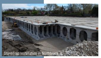
In order to prepare for the vault installation, the contractor will remove approximately 1.25 million cubic feet of soil the volume of more than 14 Olympic size swimming pools!
